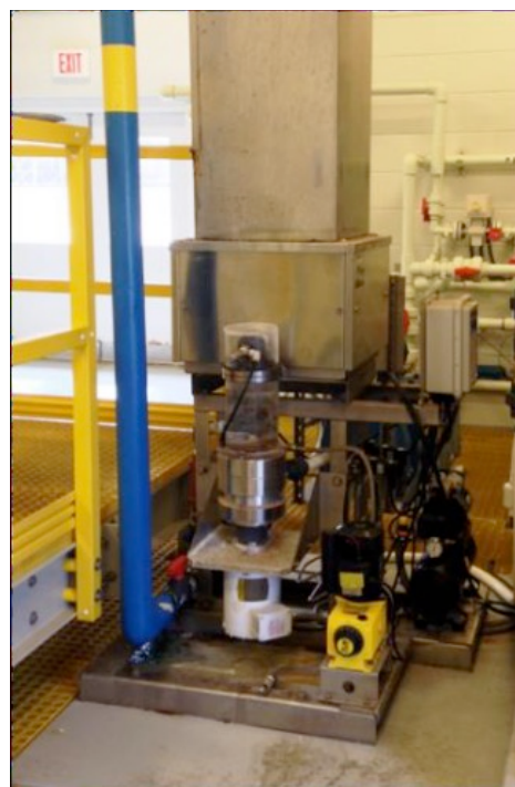
Polyblend ®DP 800 Installation at Dixon, IL
