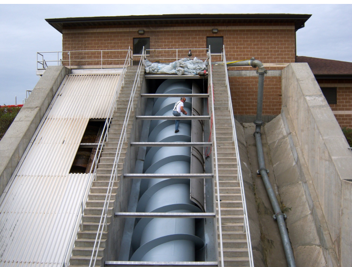
Here is one of two screw pumps located at the wastewater treatment plant in Dixon.
