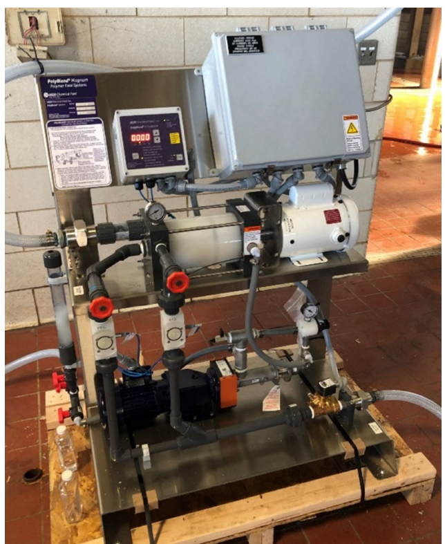
Polyblend® Demonstration Unit Installed for Testing
