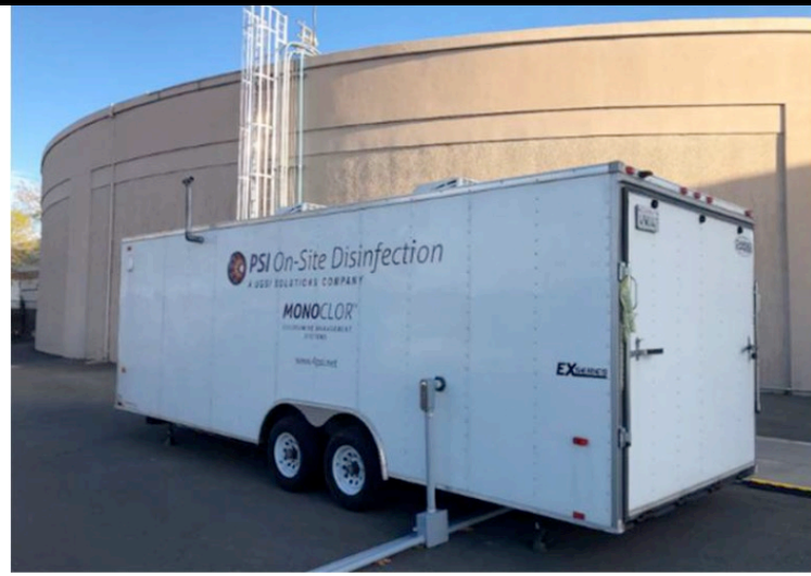
Above is the RCS trailer on site and connected to the tank
