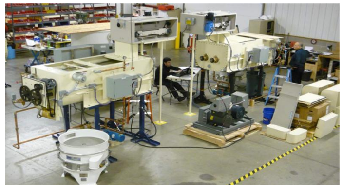
Zeeland Manufacturing Facility
