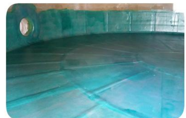
Moreno Valley Scrubber – Before/After FRP Tank Interior Refurbishment
