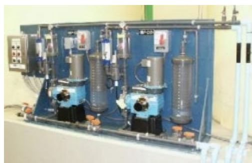
Salem, Oregon Encore® Pumps 700 metering
