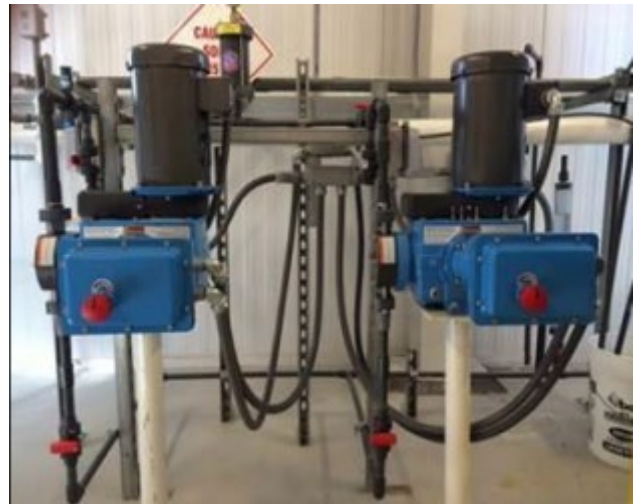
Berthoud, Colorado Clearlogx™ site where the challenge of a long pump discharge and high back pressure made the Encore® Pumps 700 an easy choice over peristaltic and positive displacement pumps
