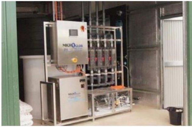
80 Pound-Per-Day (PPD) or 36 KG-Per-Day chlorine equivalent Microclor® skid, housing and proud
