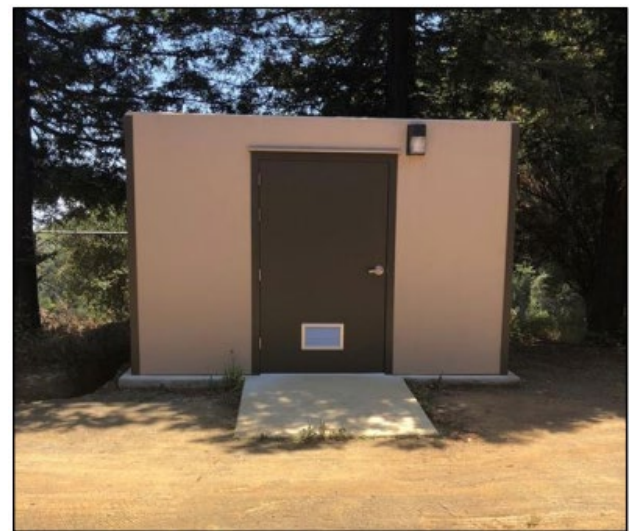
Figure 2 Neary Tank - Limited space for equipment and chemical storage
