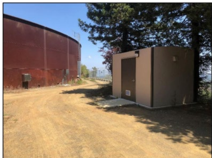
Figure 1 Neary Tank's remote hillside location
