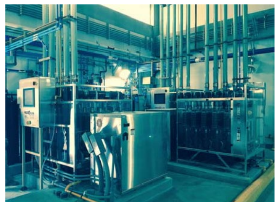
Three 1,500 PPD Microclor® OSHG skids
