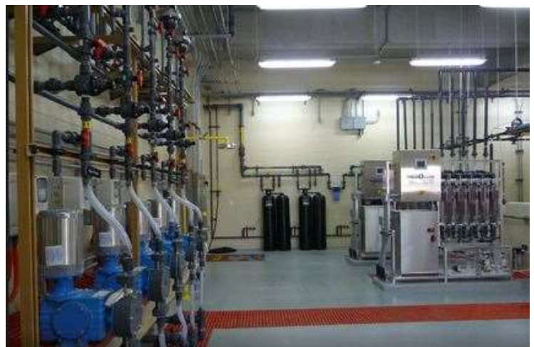
Microclor® OSHG systems with Encore® metering pumps in foreground
