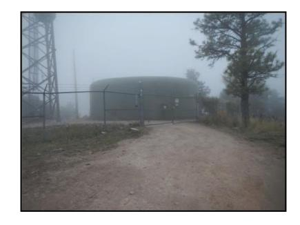
Once the THMs in the water were exposed to the air-water-interface, the Powervent® reduced the build-up of THMs in the headspace of the tank to nearly zero by continually exchanging fresh air from the tank exterior with THM-laden air within the tank. By maintaining a very low THM concentration in the tank headspace, the driving force for mass transfer of THMs from liquid to gas phase was maximized allowing for highly efficient THM volatilization.
