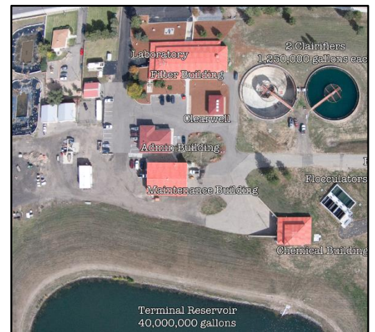
Northglenn Water Treatment Plant and the terminal reservoir
