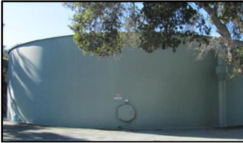
Figure 2. The Ryan Ranch tank is a 500,000 gallon steel ground storage tank
