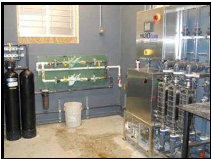
PSI Water Technologies, Inc.'s Microclor® MC-60 On-Site Hypochlorite Generation System
