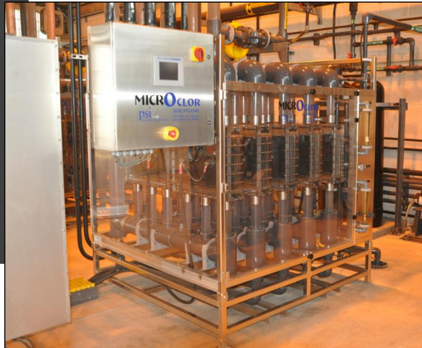
One of three 2,000 PPD Microclor® OSHG skids
