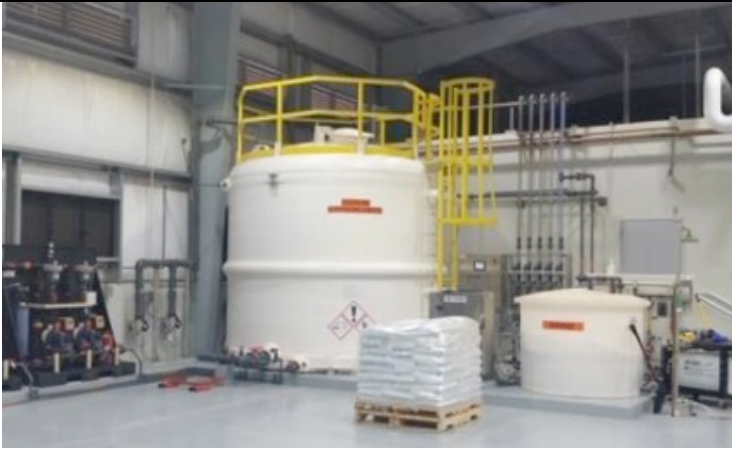
DSW Hypochlorite storage tank, brine tank and pallet with bags of salt.
